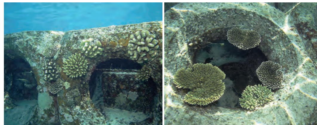
Figure 129. Natural recruitment on the surface of SHED blocks, 3.5 years after deployment in Galu Falhu. Source: Alasdair Edwards
