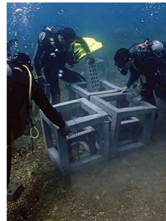
Figure 135. Divers deploying concrete blocks of different sizes in Bali, Indonesia. Source: Coral Reef Care ( https://www.coralreefcare.com/projects/ )
