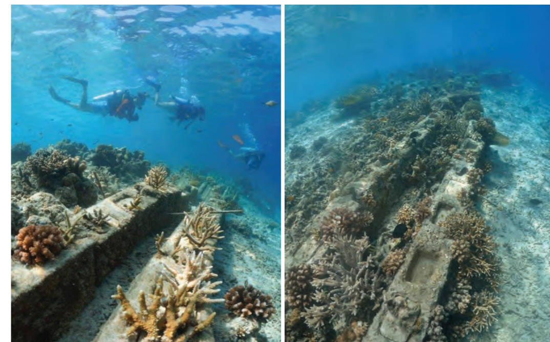
Figure 130. Concrete blocks first deployed on a reef crest in 2018-2019 (left) and after 4-5 years in 2023 (right). Source: Robin Philippo, TRACC Borneo
