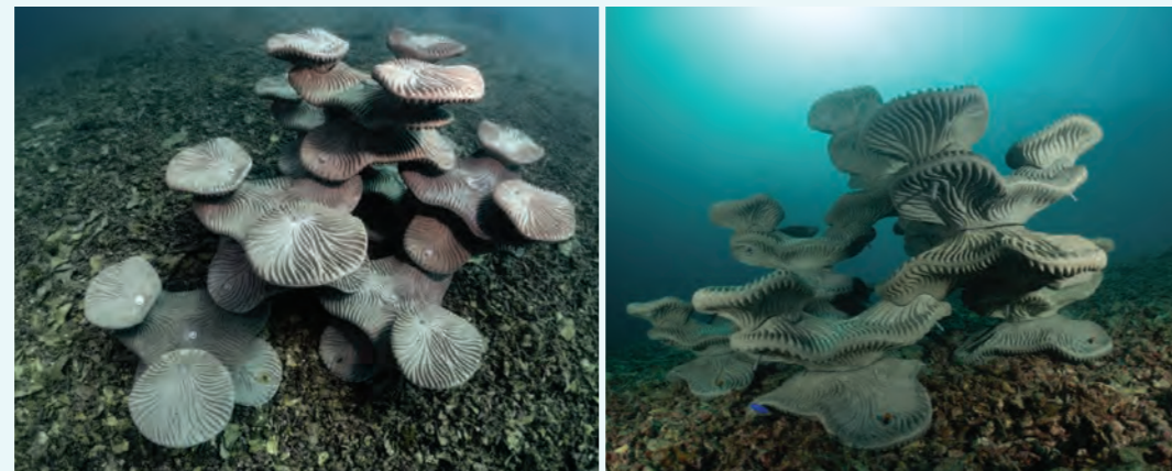
Figure 84. Photos of MARS2.0 (Reef Design Lab) deployed on a 25° rubble slope on Pom Pom Island with TRACC Borneo. Source: Robin Philippo, TRACC Borneo
