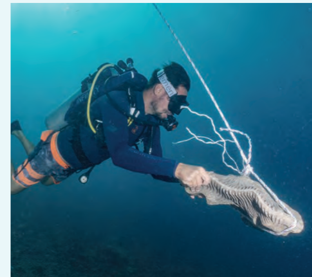
Figure 85. Diver transporting an individual MARS2.0 module for assembly at the site. Source: Robin Philippo, TRACC Borneo
