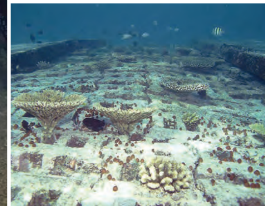
Figure 136. Armorflex mattress anchored with flooring slabs, 3.5 years after deployment in Galu Falhu. Source: Alasdair Edwards
