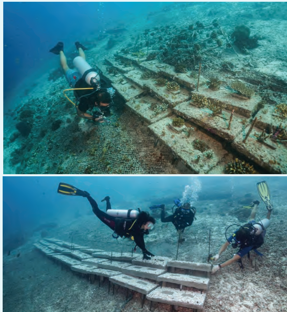
Figure 128. The revised design of step reef units, initially installed on Rugged Reef in Pom Pom Island (top), and their condition one year after installation (bottom). Source: Jeethendra and Robin Philippo, TRACC Borneo
