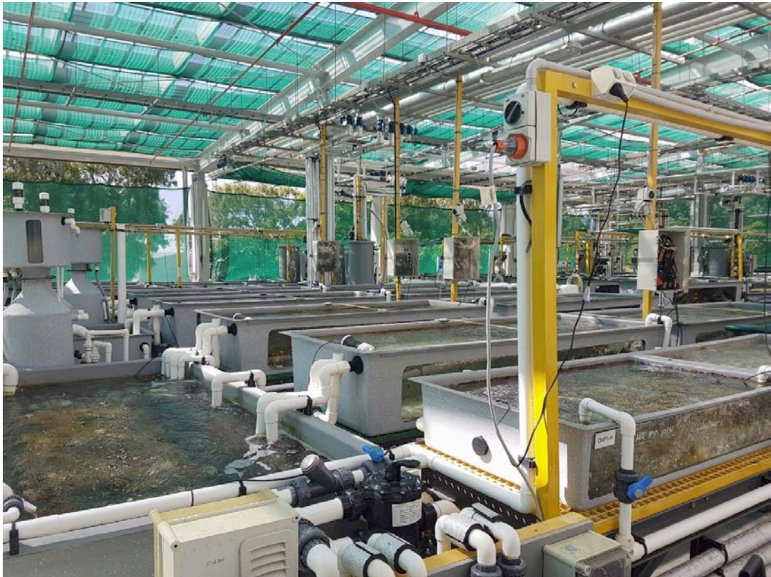
Figure 4-6: AIMS Townsville, SeaSim Open Plan External, showing holding and rearing tanks under translucent roofing.
