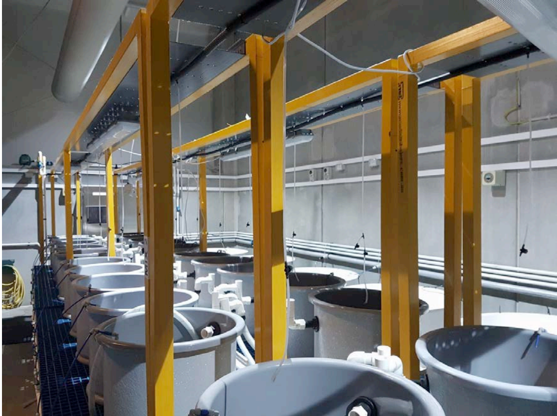
Figure 4-5: 70 litres larval rearing tanks in SeaSim. See Figure Appendix A-9-4 for 500 litres tanks for stock cultures. The proposed larval tanks are designed around the same principles, with 1400mm diameter, and 900 litres volume.
